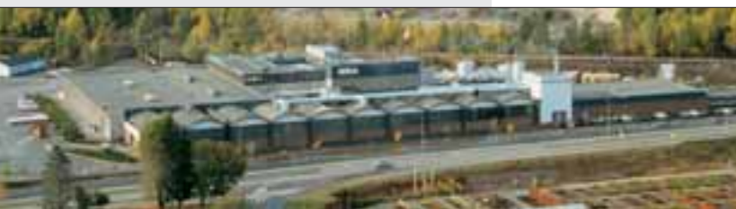
Isola Factory, Eidanger, Norway
