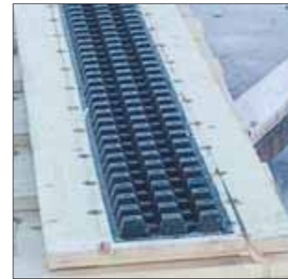
The Platon product fixed on the prefabricated form.
