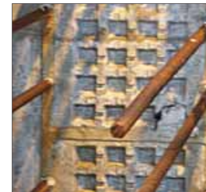
The sidewall of the box in a balanced cantilever bridge, clearly show the denticulation between the reinforcement bars.
