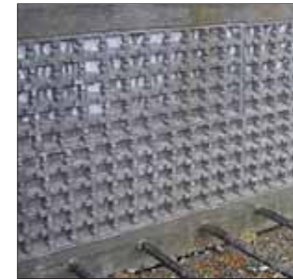
After removal of the formwork.
