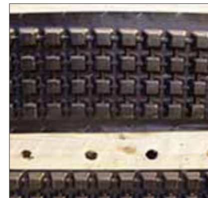
A simple and quick installation of the sheet at the form.
