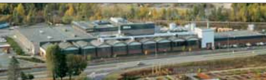
Isola Factory, Eidanger, Norway
