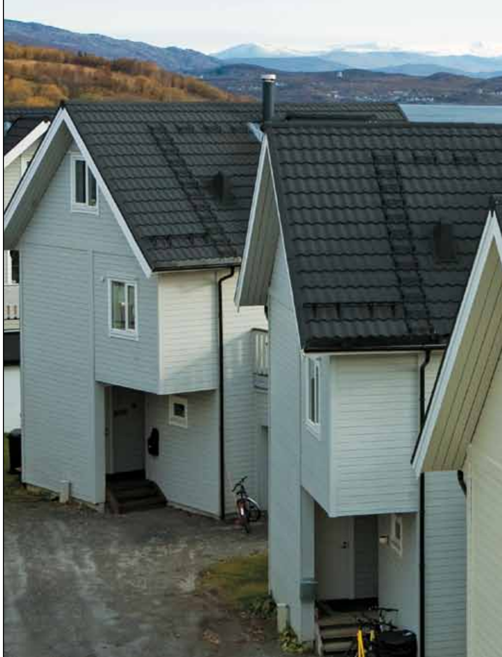
People in Norway know how to protect their house against wind and weather.
