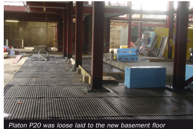
Platon P20 was loose laid to the new basement floor
